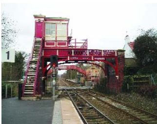
Wylam Signal Box
